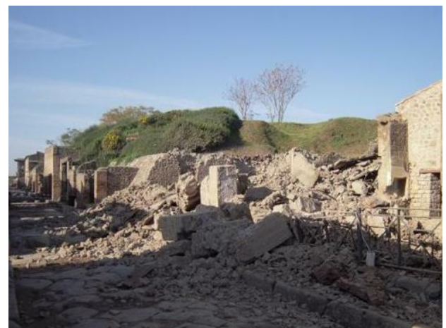
Figure 4. Archaeological site of Pompeii. Schola Armaturarum after the collapse.
