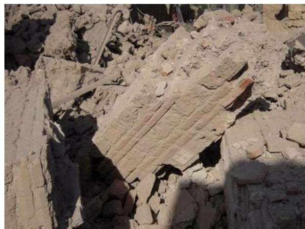
Figure 5. Archaeological site of Pompei. Schola armaturarum. Detail of the collapsed masonry.
