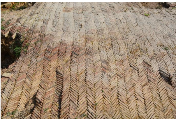
Figure 5: Opus spicatum floor in the unit C.
