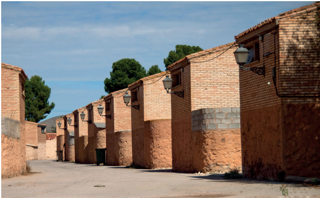
Figure 7. Cañada de Agra. Traffic alley.
