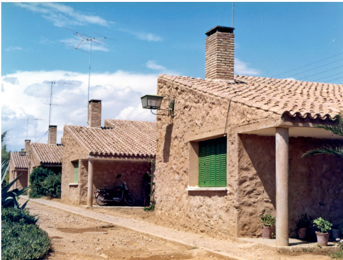
Figure 6. Cañada de Agra. Pedestrian way.
