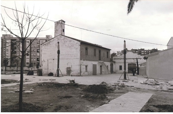
Fig. 4. Image of the original condition of the factory. (Source: V. Algarra, P. Berrocal, archaeological report, 2001)
