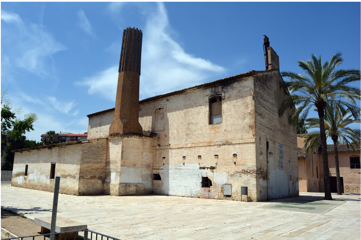
Fig. 1. Image of the previous condition of the factory. (Source: the authors 2018).
