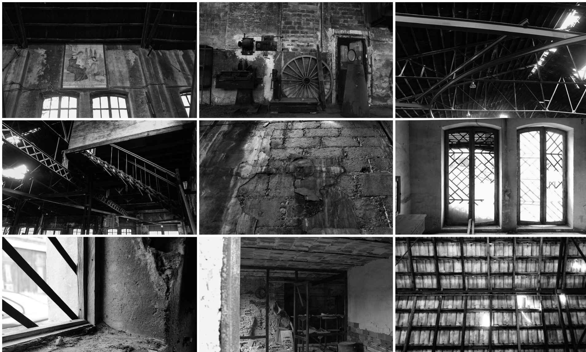
Fig 23. Taller dels Canets (former San Antonio wooden carriage factory), Beneixama (Alicante, Spain), January 2021. Interior photographs in detail of the workshop initial state before measurements and drawings were made. Materials, texture, surfaces. (Ortin Molina, S.; Ortin Molina, M. A., photographs and digital image post-editing work).
