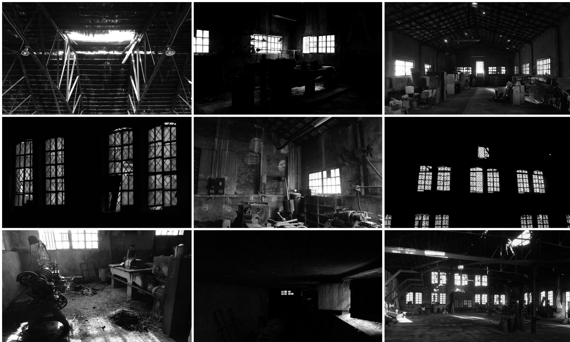
Fig 21. Taller dels Canets (former San Antonio wooden carriage factory), Beneixama (Alicante, Spain), January 2021. Interior photographs of the initial state of the factory before measurements and drawings were made. Workshop spaces: risks and hope. (Ortin Molina, S.; Ortin Molina, M. A., photographs and digital image post-editing work).
