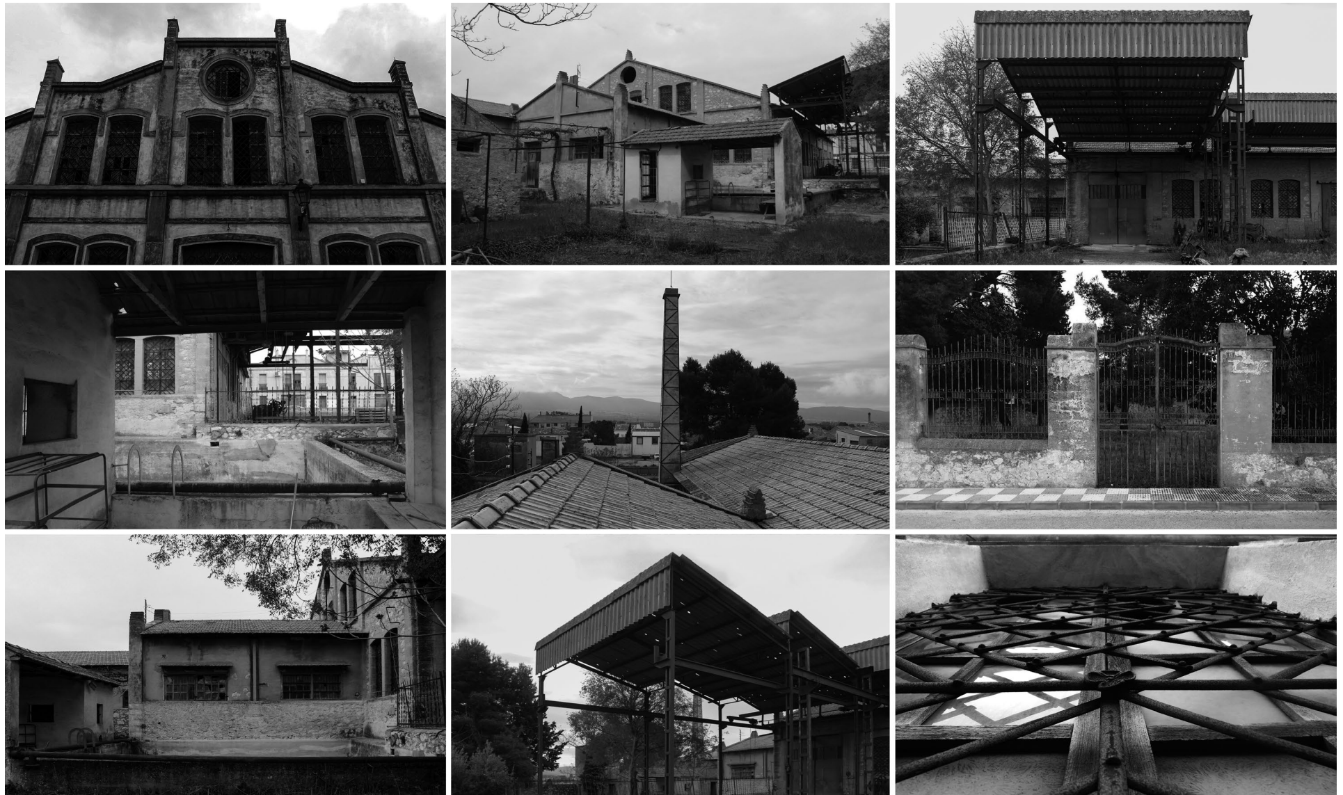
Fig 22. Taller dels Canets (former San Antonio wooden carriage factory), Beneixama (Alicante, Spain), January 2021. Exterior photographs of the initial state of the factory before measurements and drawings were made. Façades, porchs, raft and terrace. (Ortin Molina, S.; Ortin Molina, M. A., photographs and digital image post-editing work).
