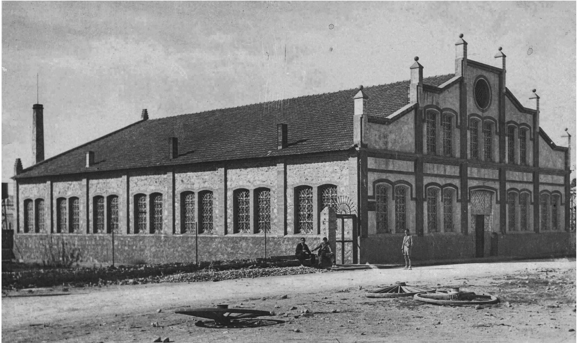
Fig 1. Taller dels Canets (former San Antonio wooden carriage factory), Beneixama (Alicante, Spain), 1930-1940. Historical photograph of the carriage factory before the construction of the outer porch at the east terrain and the attached warehouses. (Stock image courtesy of S. Sanchis, one of the current owners of the Taller dels Canets).
