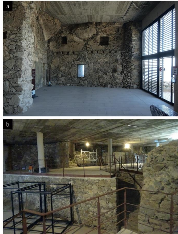
Figure 5: The fort. Interior. Current state and details of the walls that show the presence of different levels, arches, etc.: a) First floor; b) basement -1 (Arxiu Didpatri-UB).
