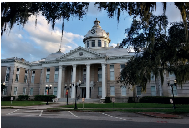
Fig. 3. The OPCC building. (Source: authors).
