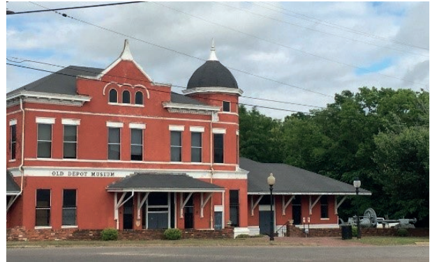
Fig. 4. The ODM building. (Source: authors).
