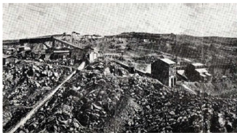
Fig. 2. Building works in Esla Dam, 1932 (Source: Saltos del Duero, 1933).
