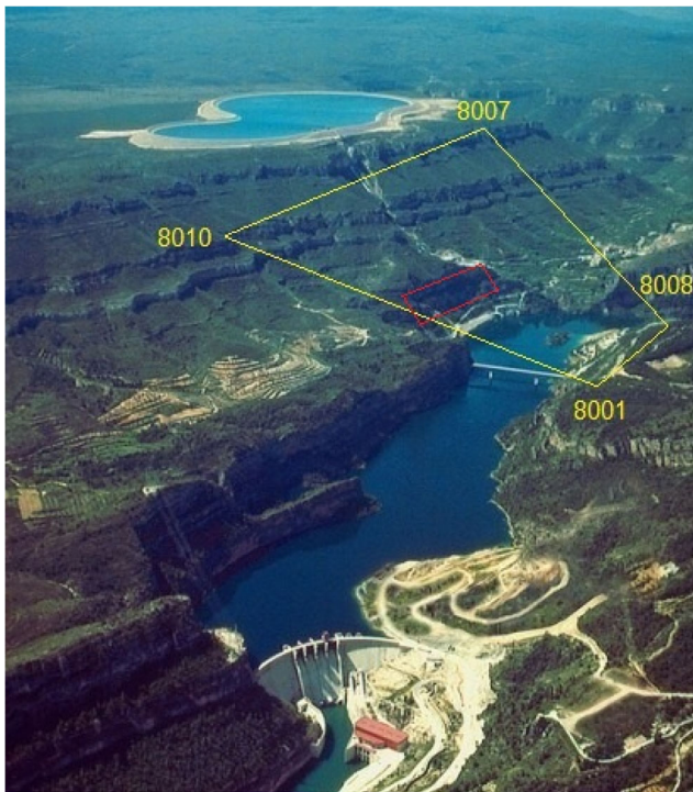
Fig. 1 Overview of the electricity power complex in Cortes de Pallás. The four extreme pillars of the geodetic network are sketched in yellow (8001, 8007, 8008, 8010), and the critical area to be monitored is framed in red
