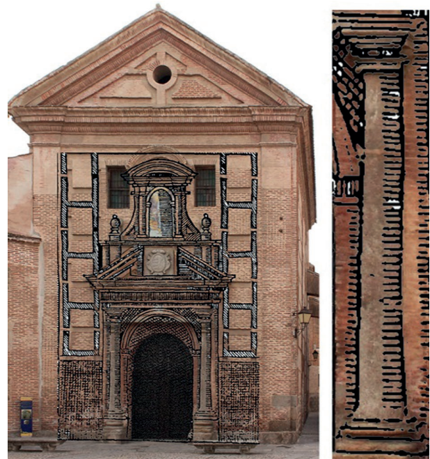
Fig. 3. Convent of the Madres Bernardas de la Encarnación. Montage superimposing Fray Lorenzo's tracing on the rectified image of the building's façade, in which the coincidences referred to can be seen. In both images the real proportions of the drawings of the treatise have been respected. Source: Composition by authors.
