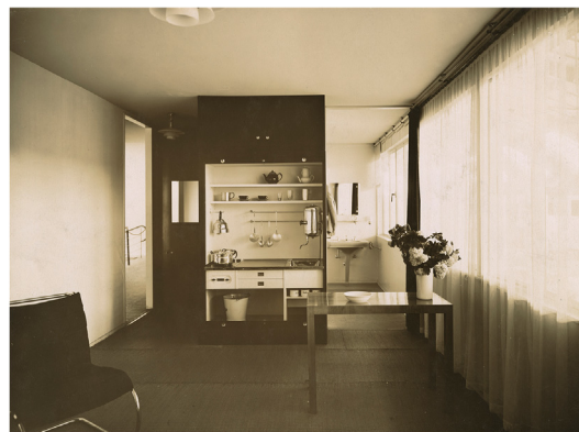
Fig. 9 Cooking cabinet. The Dwelling in our Time Exhibition. Lilly Reich, Berlin, 1931. Source: Ludwig Mies van der Rohe Archive, The Museum of Modern Art, New York.
