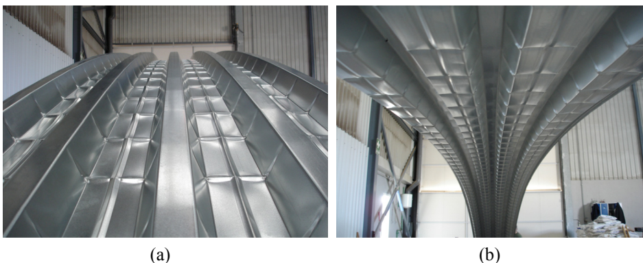
Figure 1: (a) Superior and (b) inferior views of a cold-formed arch. Rolling process provides the crests and valleys in the sheeting. Hammering effect is seen in the folds.
