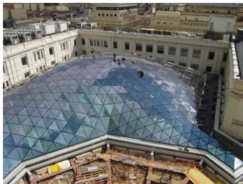
Figure 11: Aerial view of the finished structure with glass
