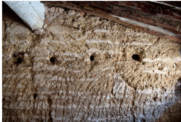
Figure 4. Detail of the interior surface of the earthen wall on the upper level of the dwelling. Source: L. Balaguer.
