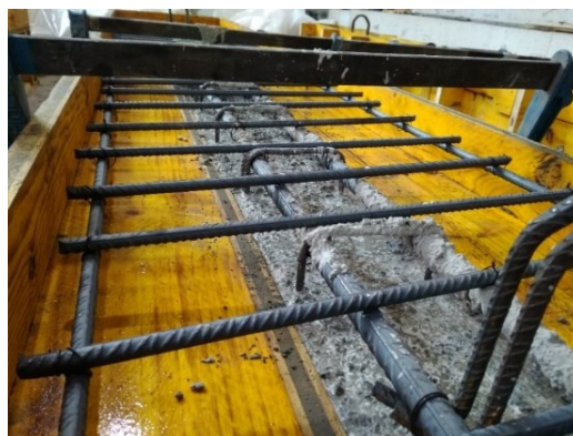
Fig. 4. “As cast” interface appearance before the cast-in-place slab’s concrete casting.
