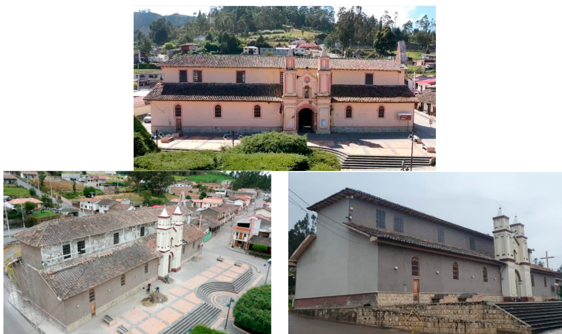
Figure 16. Monitoring of the Nabón Central Church. Status of the church in March 2021 (top), August 2021 (bottom left), and November 2021 (bottom right).
