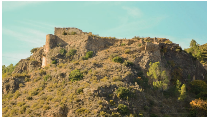
Figure 7. Domeño Castle, an example of a rock fort adapted to defend the road to Chelva.
