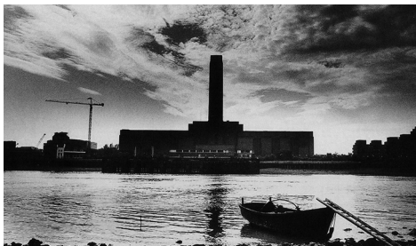
Fig.3.31. Bankside Power Station en 1989.
