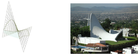
Figure 4 Left: One hyper generating form for Chapel Lomas de Cuernavaca Right: Chapel Lomas de Cuernavaca (Mexico, 1951) [5]
