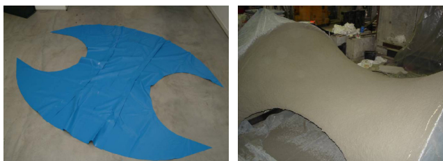
Figure 2 Left: Fabric formwork assembled for the double-curved shell. Right: Resulting concrete shell
