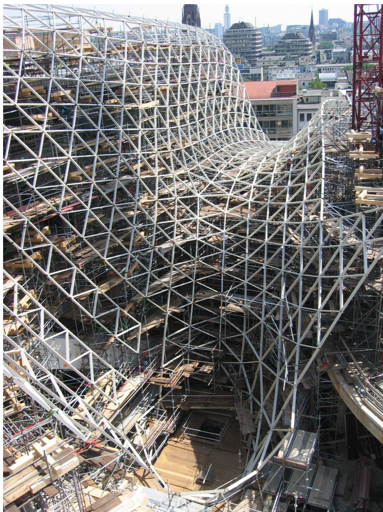
Figure 11: grid during construction
