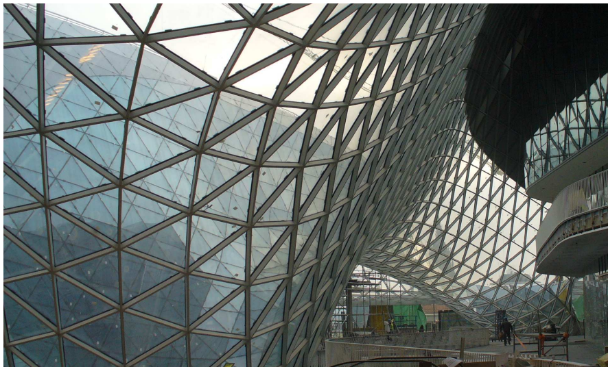
Figure 12: grid during construction
