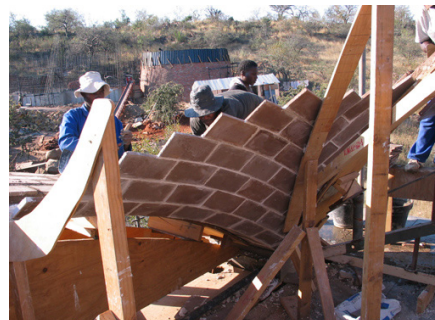
Figure 6: Tile vault construction requires only geometric guides
