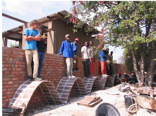
Figure 9: Test Vaults built on site
