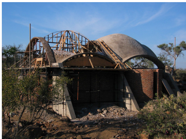
Figure 8: Wooden guides established the geometry
