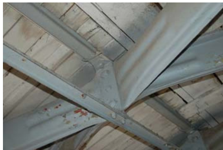
Figure 7: C-shaped lamella with stiffening corrugations and normal screws, probably standard design since 1930
