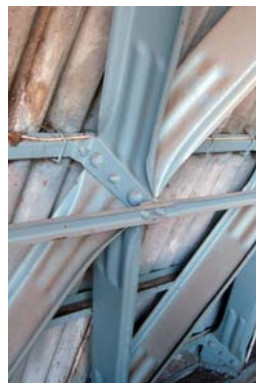
Figure 4: Joint System Junkers
