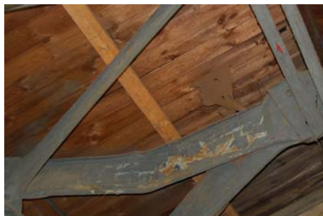
Figure 11: Boathouse Dessau, erected 1930 Figure 12: damaged lamellas after a bomb hit in 1945; situation 2008
