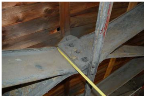
Figure 6: S-shaped lamella without corrugations and hole screws, probably standard design till 1930
