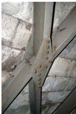
Figure 3: Joint System Huennebeck
