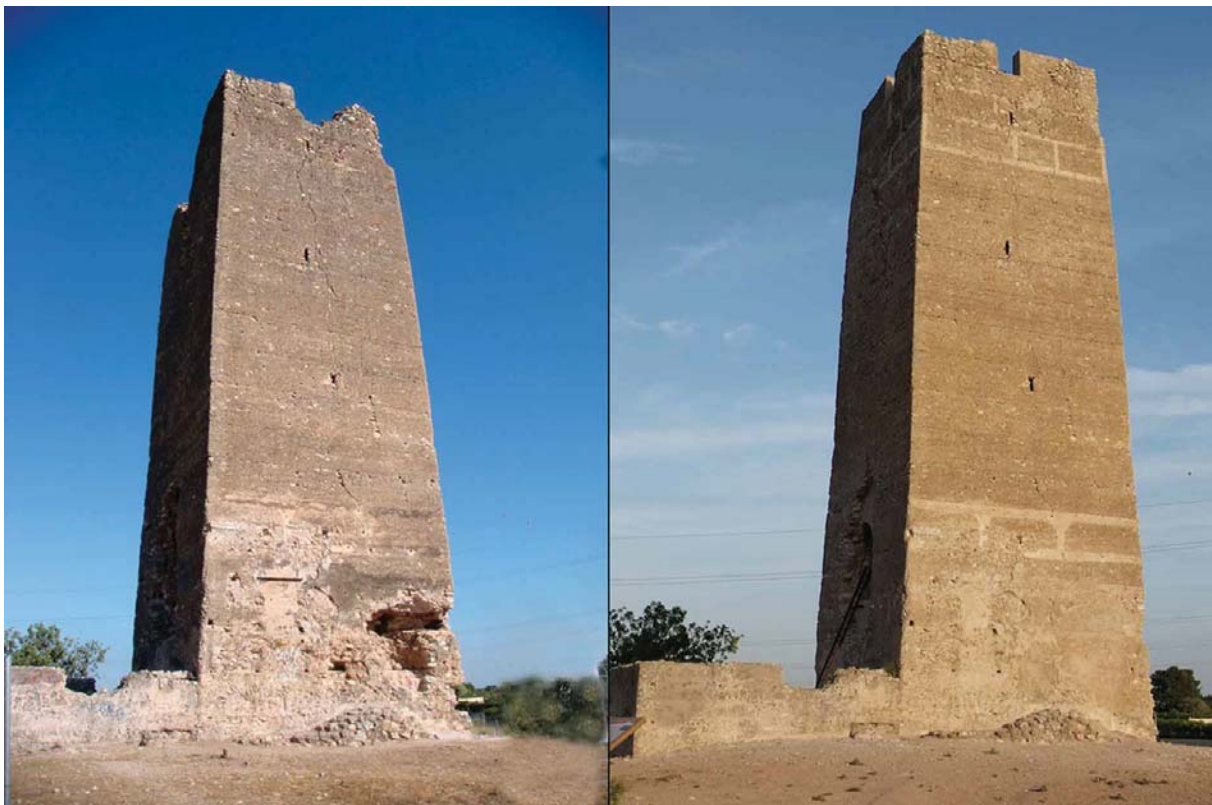
Figure 6. The tower, after and before preservation works (Cristini).
