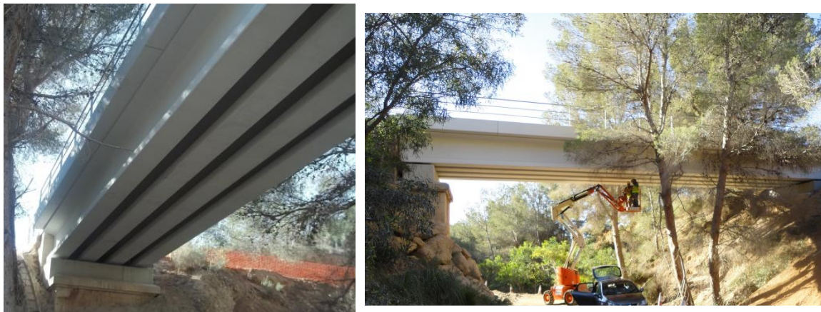
Figure 7. The Moneder Gully Bridge.
