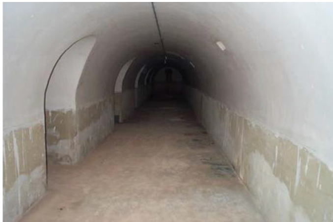
Figure 2: Air-raid shelter in Luis Vives high school.
