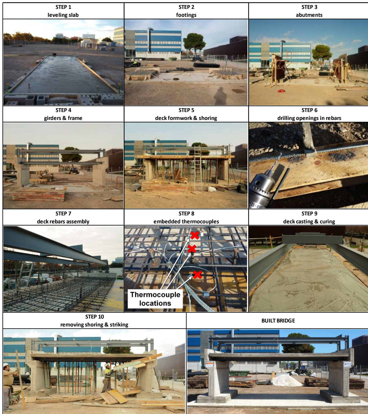
Figure 2. Construction process of the experimental bridge.
