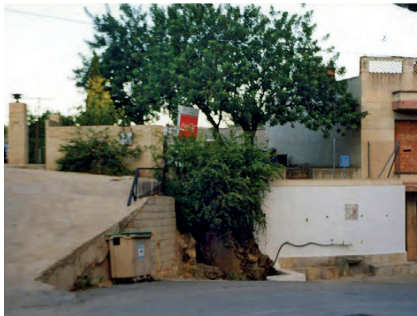
Figura 3. Estado original (1999) / Figure 3. General view before work started (1999).
