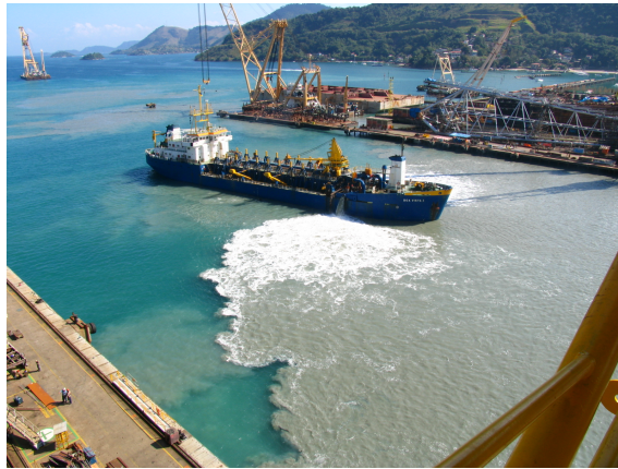
Figure 2.2: Example of water pollution in a port. 2
