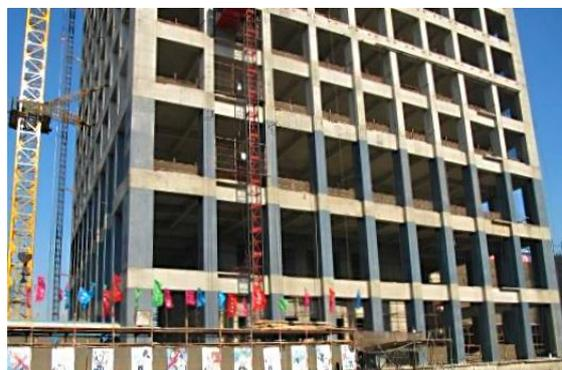
Fig. 1. A buildings using STCRC columns in the bottom three stories [1]
