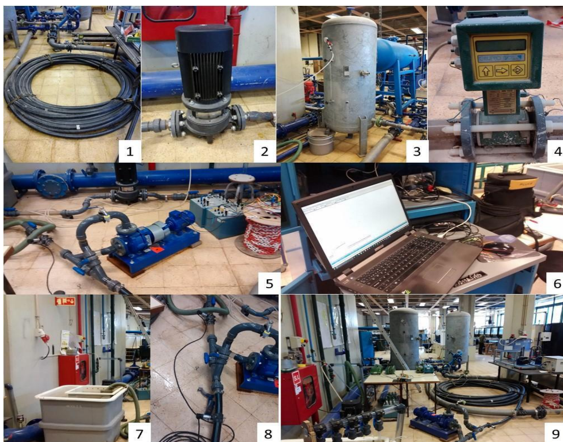
Figure 5. Components of the experimental facility: (1) HDPE pipe; (2) recirculating pump; (3) air-vessel tank; (4) flowmeter; (5) PAT; (6) picoscope and acquisition data; (7) downstream regulating tank; (8) pressure transducers and (9) general view.
