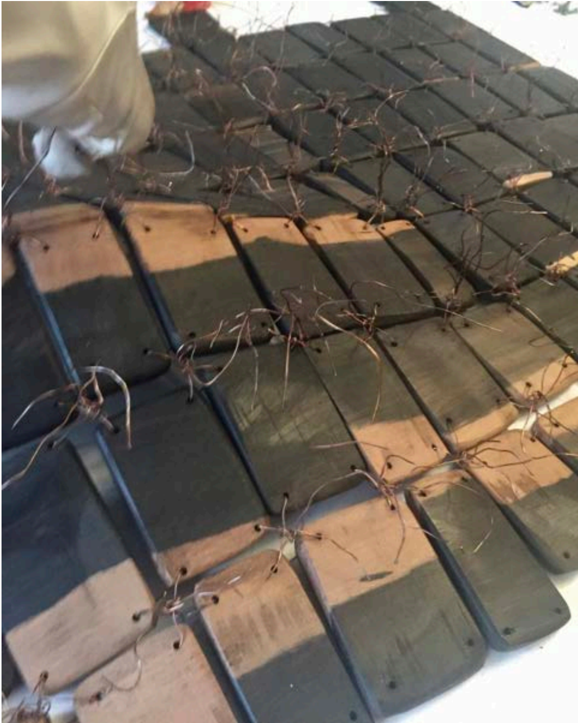
Image 44. Work in Progress. 2016
