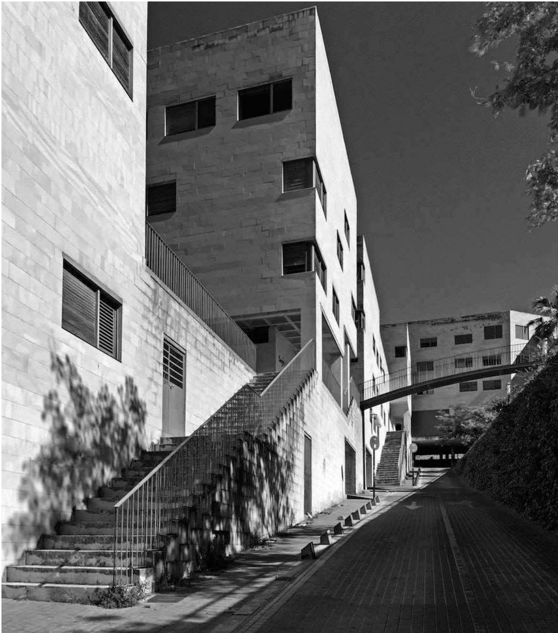
Figure 6. View of La Sang ramp, in the neighborhood of La Sang, by Manuel de Solà-Morales
