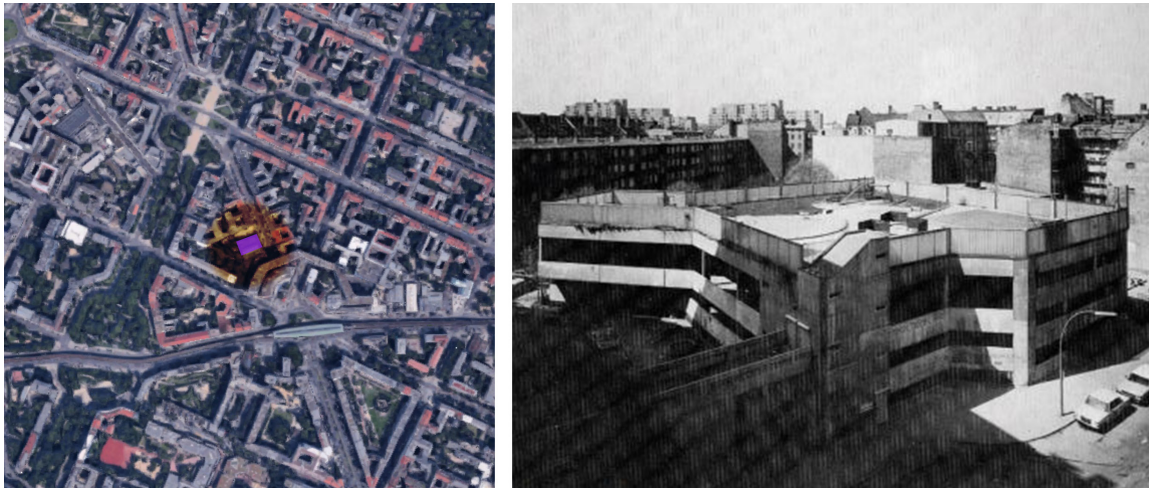
Figure 1. The INA kindergarten is at the east part of the Kreuzberg in Berlin (left). The exterior of parking garage prior to the conversion (right).
