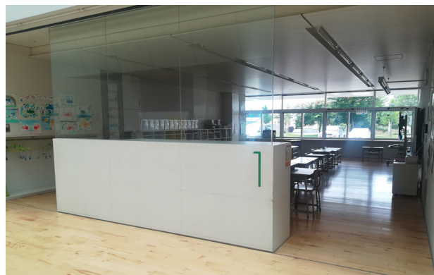
F131 Transition between classroom and multi-purpose space in Numata Elementary School.
