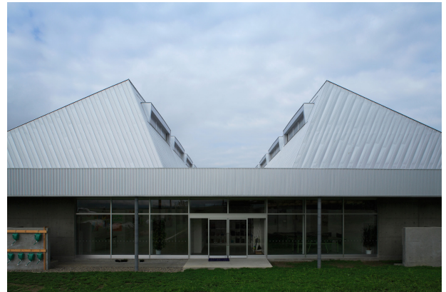
F119 North-South façade.
