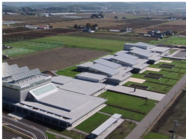
F135 Higashikawa Elementary School.
