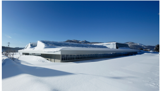
F108 Image from the exterior of the school during winter.
