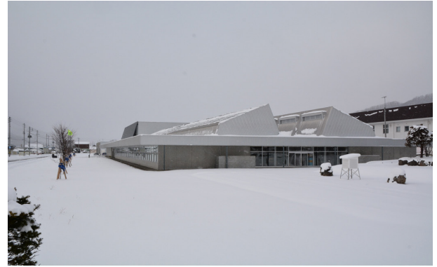
F107 Image from the exterior of the school during winter.
