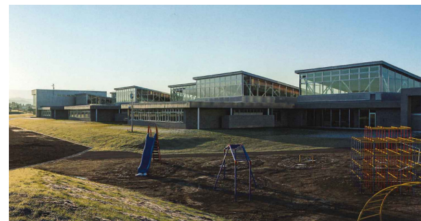
F136 Higashikawa Elementary School.
