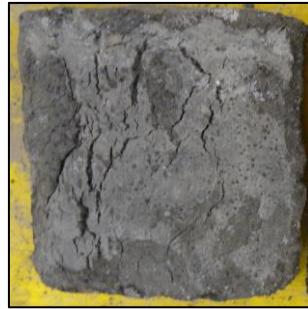
Figure 45. Cracks due to deformation (1)
