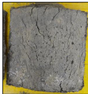
Figure 46. Cracks due to deformation (2)
