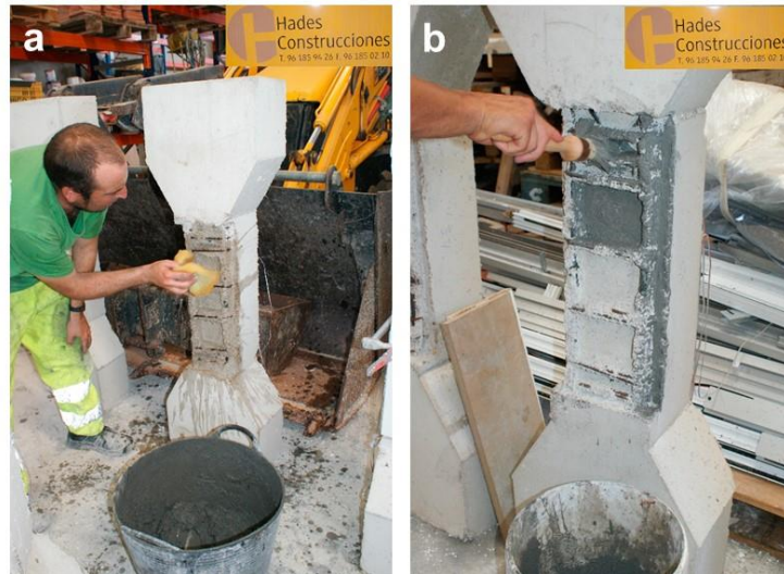
Fig. 3. a) Dampening the surfaces; b) Applying the binder.
