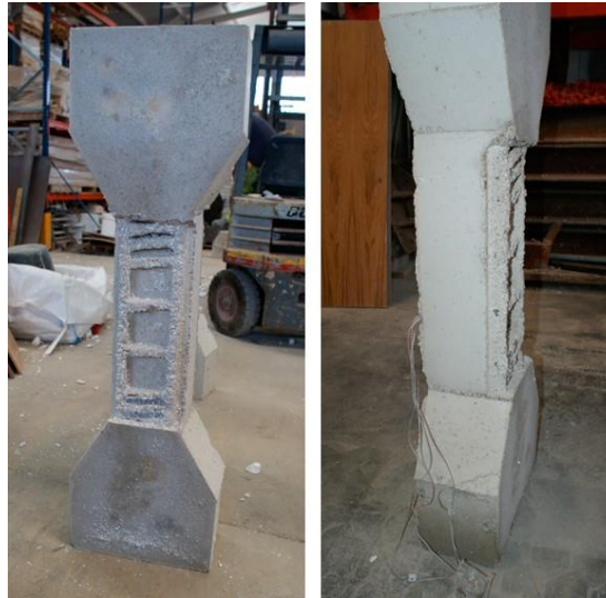
Fig. 2. Damaged Column before being repaired
