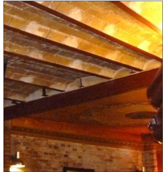
b. Rolled steel joist and beams
