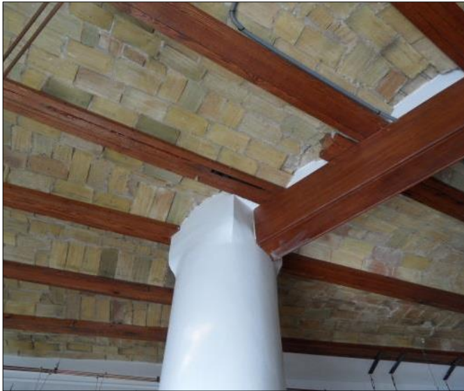
a. Timber joists and beams
