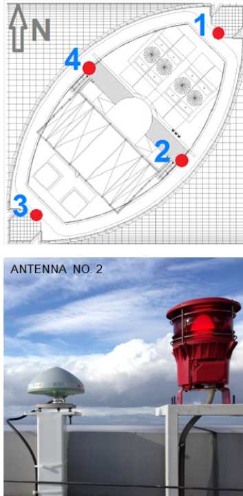
Figure 2: Building Torre Espacio, Madrid. Four GNSS antennas on rooftop
