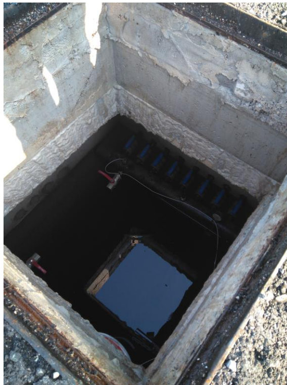
Figure 2.17. Collector pit of the BHE field
