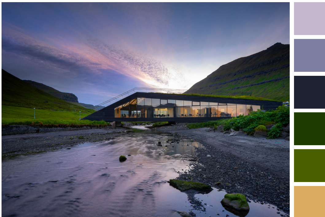
Fig. 42 Seen here the blending of the project with the colors of nature around
