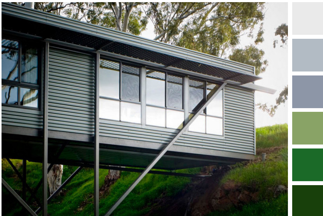
Fig. 41 Façade detail and contact with the ground. Max Pritchard Architect
