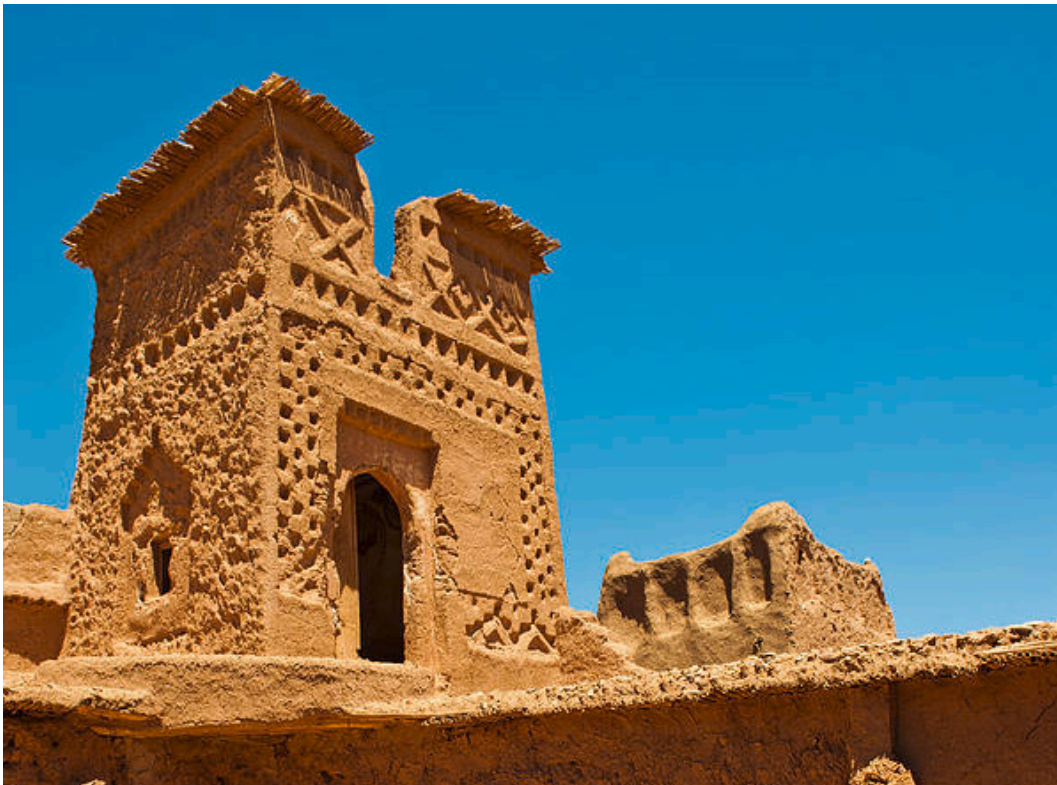
Fig. 2 - Deatil of one of the towers and the ornamentation made of clay
