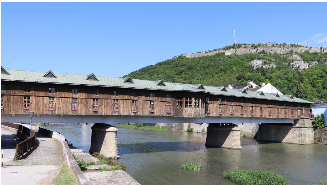
Fig. 9 - Image of the newest covered bridge, with metal beam support.
