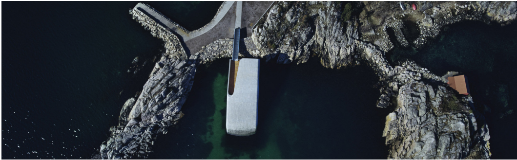
Fig. 68 Landscape setting of the project
