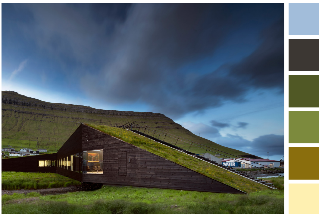
Fig. 44 Building rising from nature from the sides. Creates a community meeting area
