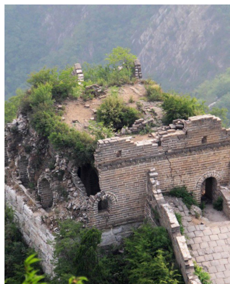
Fig. 12 - Degradation when nature takes over
