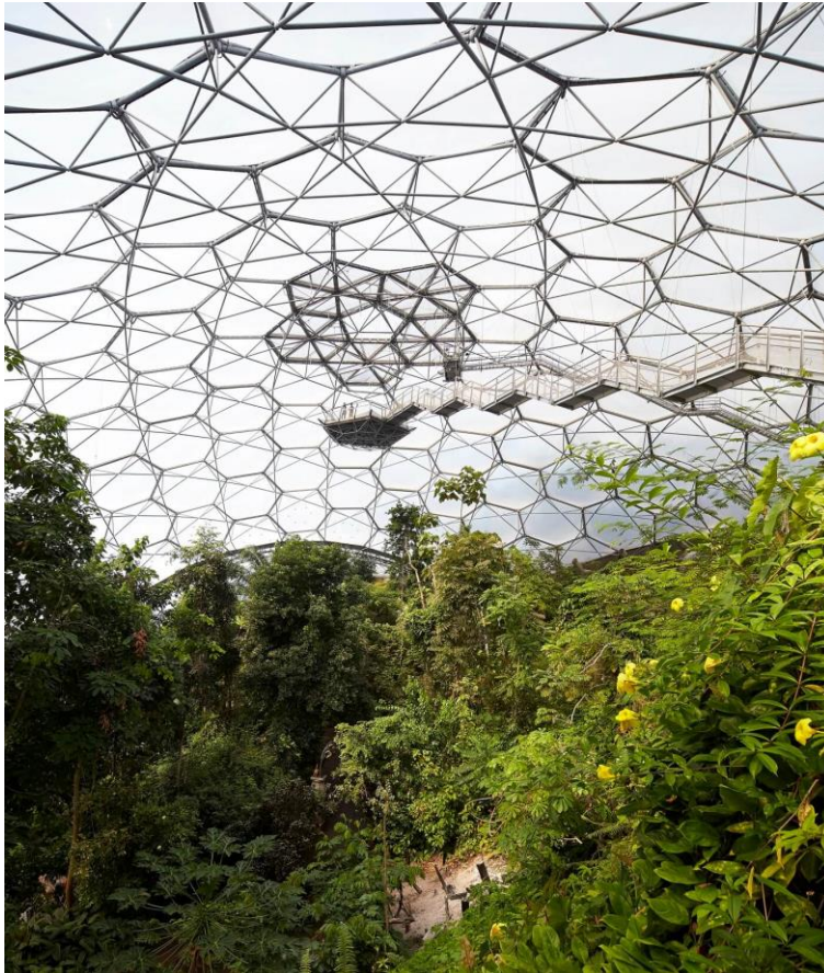
Fig. 70, Vista interior Eden Project
