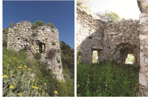
Fig. 8. Southern tower near Sykia channel (Simou, 2019).
