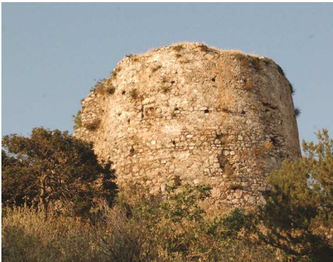
Fig. 6. Round Tower-bastion N1 (Mamaloukos, 2012).
