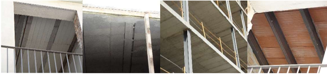
Fig. 11 Reinforce concrete and steel structures (credit: the authors)
