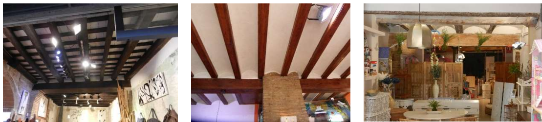
Fig. 8 URM with one-way floors, timber beams and joists (credit: the authors)
