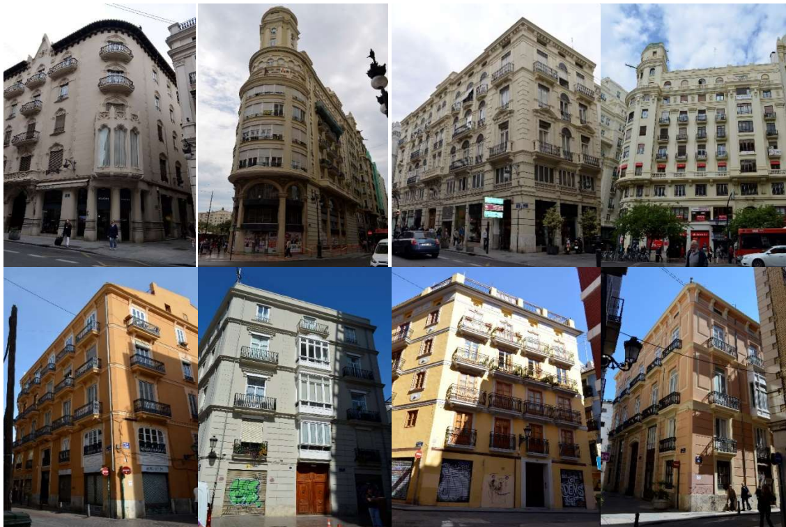
Fig. 18 Buildings in Ciutat Vella with the highest vulnerability indices (credit: the authors)
