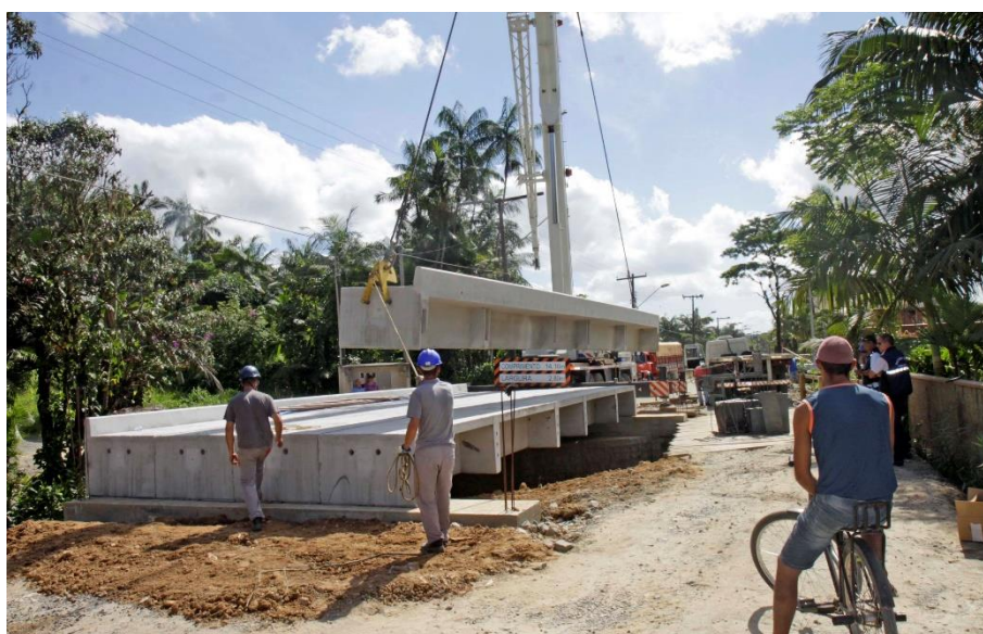
Figure 18. Obstacle transposition kit over Motucas River, at Estrada dos Portugueses, Vila Nova neighborhood, Joinville-SC - Type P23 PMD 5V. Source: Joinville City Hall [75].
