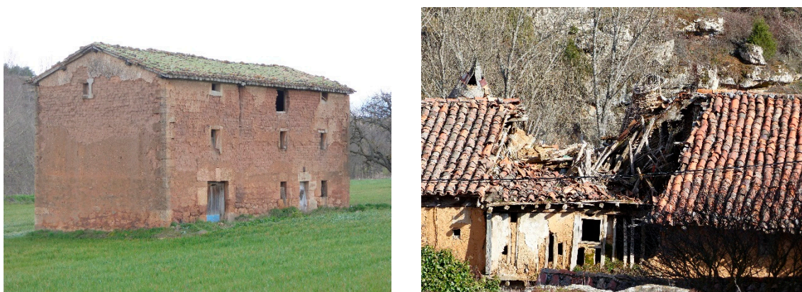
Figure 14. Abandoned constructions in areas with low population. Left: Adobe abandoned construction in Salas de Bureba (Burgos). Right: Half-timber construction collapse in Calatañazor (Soria). Source: authors.
