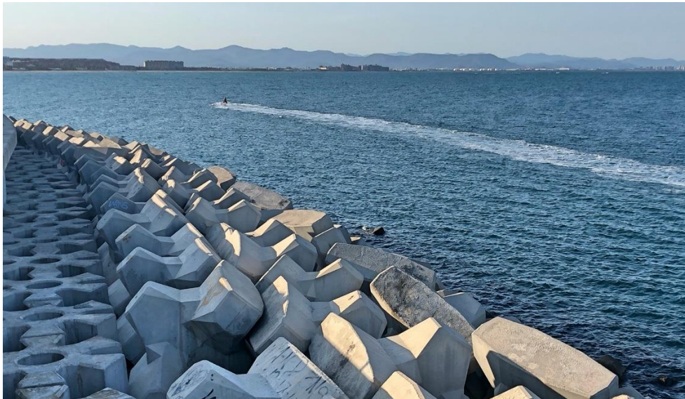
Port of Valencia (Spain), May 2020
