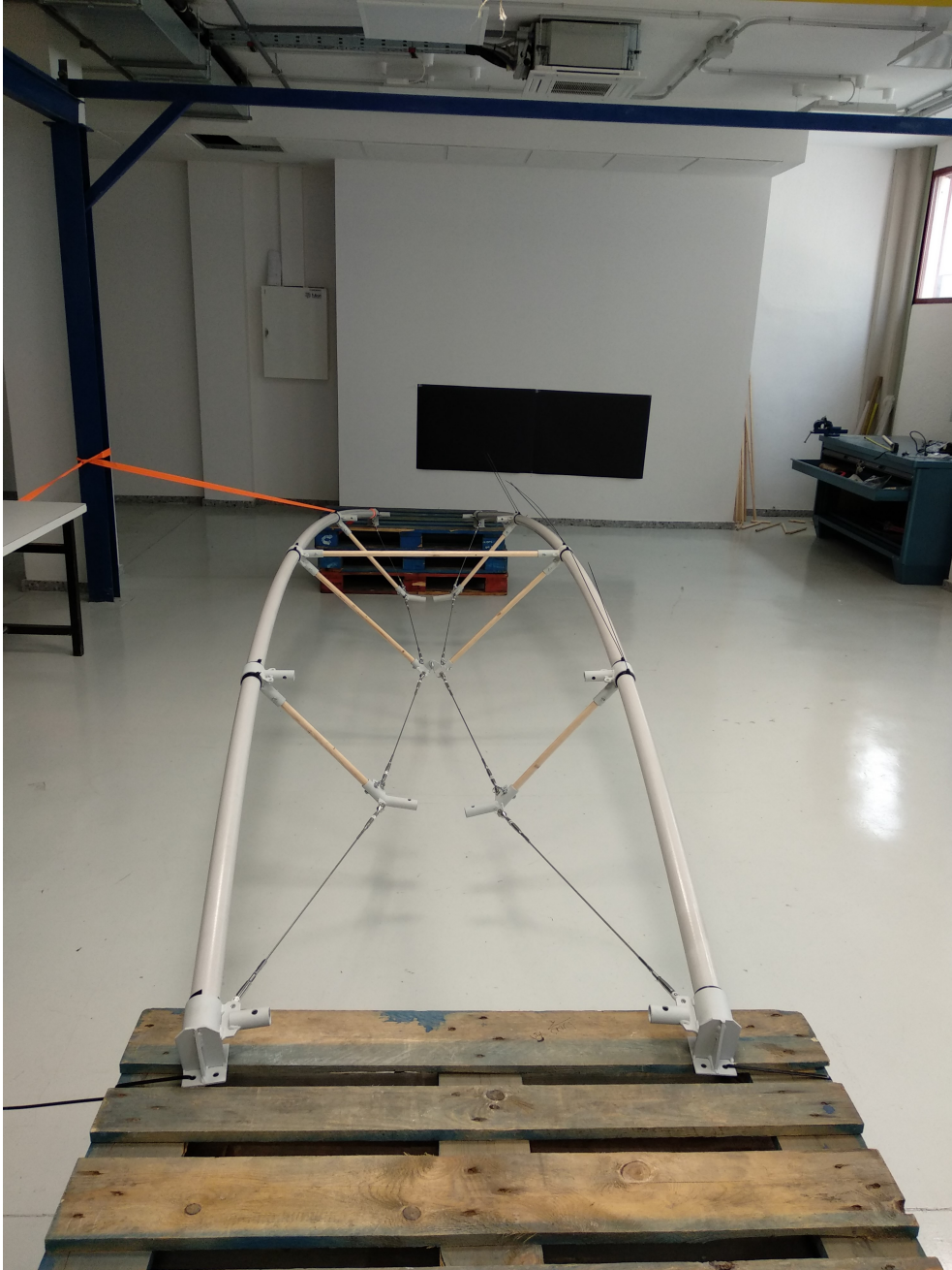
Figure 92: Erection process of the prototype (g).
