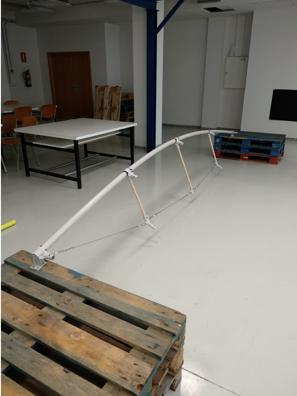
Figure 90: Erection process of the prototype (e).
