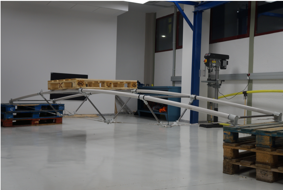
Figure 83: Experimental footbridge based on the active-bending principle.
