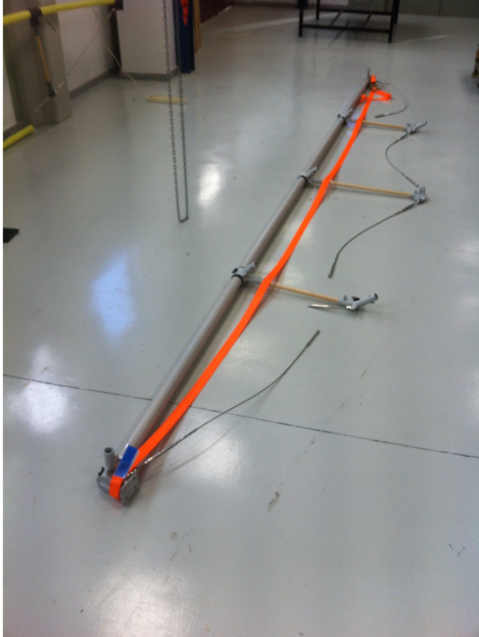
Figure 87: Erection process of the prototype (b).
