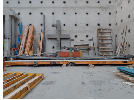
(b) Final configuration after the tensioning process.
