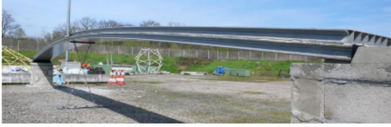
(a) Experimental footbridge using a beam prestressed by bending [12].
