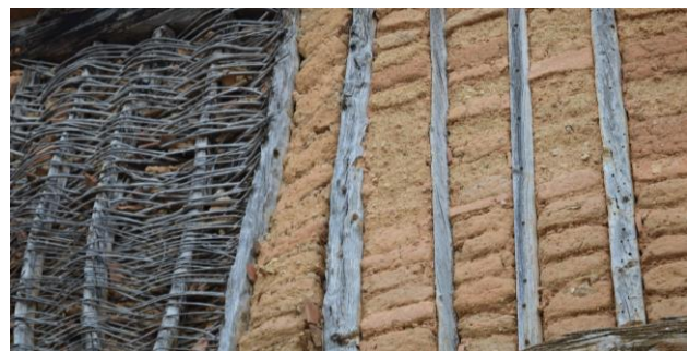
Figure 1. Half-timbered wall with wattle-and-daub (light interwoven fibres) and adobe filling (heavy masonry pieces).
