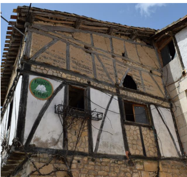
Figure 11. Building in Valdazo (Burgos), aesthetically updated with mortar rendering.
