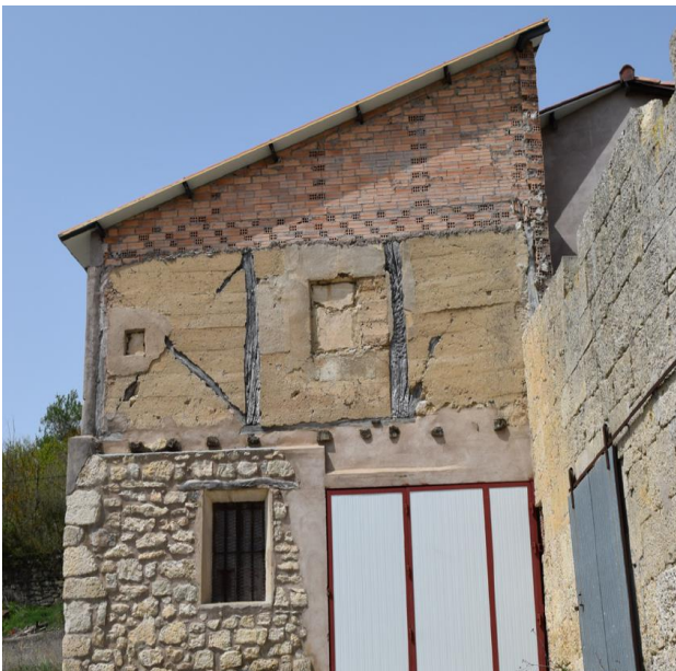
Figure 10. Building in Reinoso (Burgos), extended with brick walls and rehabilitated as a garage.
