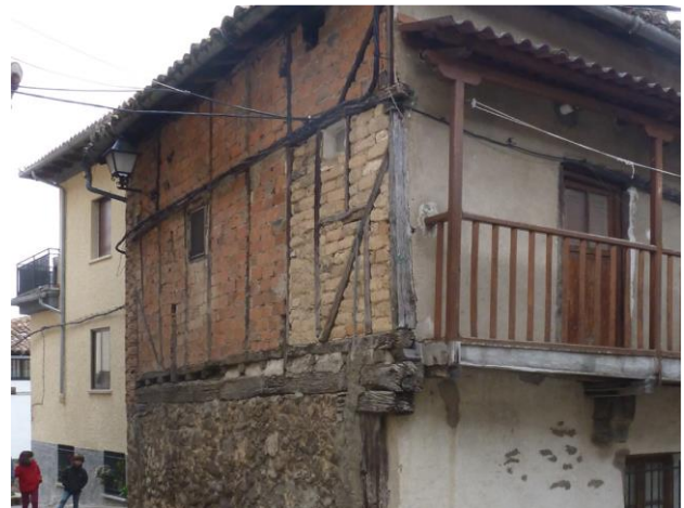
Figure 8. Building in Garganta la Olla (Cáceres), in which adobe infill has been substituted with industrial bricks.
