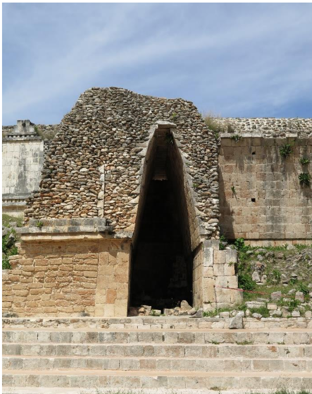
Figure 1. Vault with highly specialized vault stones in the Building 22 of the Puuc site of Uxmal (Yucatan, Mexico).
