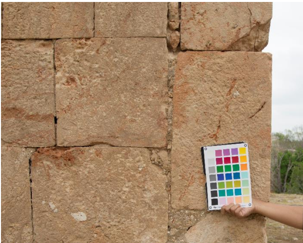
Figure 3. Using a color checker chart during the photogrammetric survey in Uxmal.
