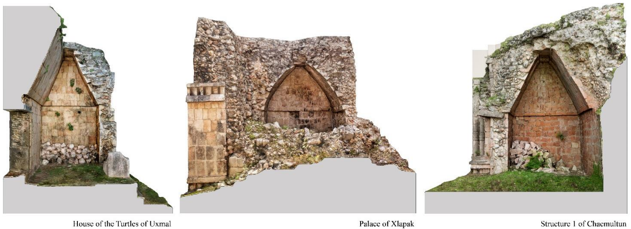
Figure 5. 3D models of three Puuc vaults obtained from the photogrammetric surveys.
