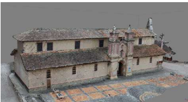
Figure 8. Nabón's church dense point cloud
